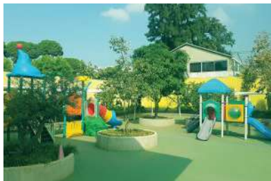
SOEURS FRANCISCAINES SCHOOL Waterproofing, concrete repair & playground
