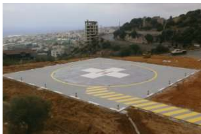
AL MAOUNAT HOSPITAL Helipad coating
