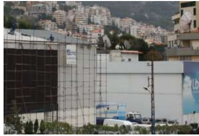
LBCI Waterproofing & insulation
