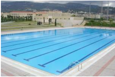
LEBANESE UNIVERSITY Waterproofing & swimming pool
