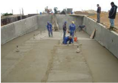
Plastering, screed, waterproofing, tiling & grouting
