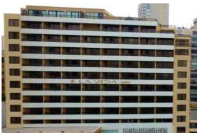
LA VIDA SUITE HOTEL Façade renovation
