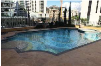
DAMAC TOWER Swimming pool & mosaic tiles
