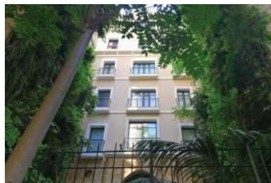
CONVIVIUM V Façade renovation
