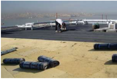
MTV Waterproofing & insulation
