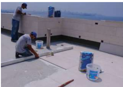
Tiling, painting, cornice installation...
