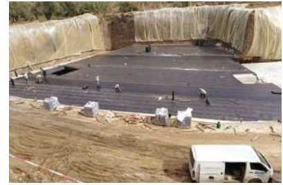
EL YOUSSEF MEDICAL CENTER Waterproofing
