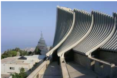
NOTRE DAME CATHEDRAL Waterproofing, concrete repair & paint
