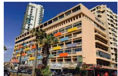
SHAMS BUILDING Façade renovation
