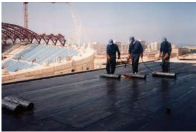
BEIRUT SPORT CITY Waterproofing & insulation
