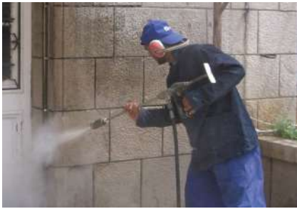
Water-jet cleaning, concrete repair, painting...
