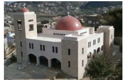
ANNUNCIATION CHURCH Waterproofing
