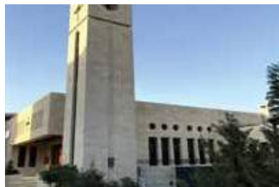
EVANGELICAL LUTHERAN CHURCH - AMMAN Waterproofing
