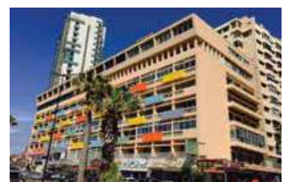
SHAMS BUILDING - BEIRUT Façade renovation
