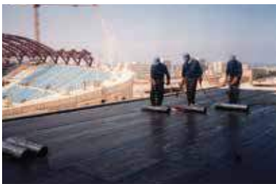
BEIRUT SPORT CITY - JNAH Waterproofing & insulation
