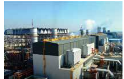
BESMAYA POWER STATION - BAGHDAD Floor coating & sealants
