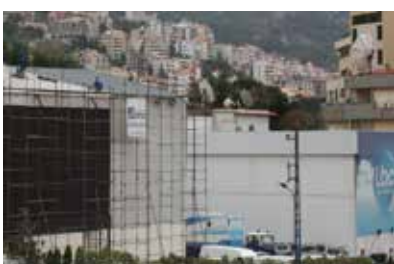
LBCI TV STATION - ADMA Waterproofing & insulation
