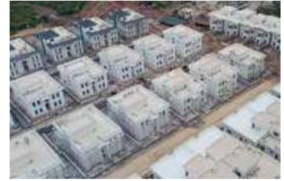
FRENCH VILLAGE - DOHUK Waterproofing
