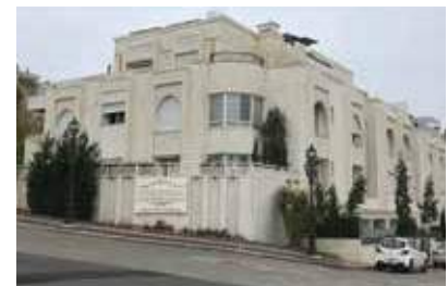
CORDOBA COMPOUND - AMMAN Waterproofing
