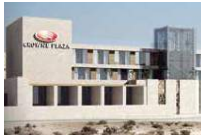
CROWNE PLAZA HOTEL - AMMAN Waterproofing
