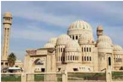
GRAND MOSQUE - MOSUL Water-repellents
