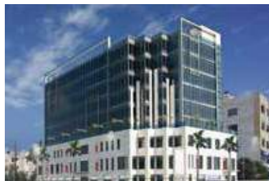
ABU RAKHIEH PLAZA - AMMAN Waterproofing
