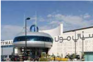
CITY MALL - AMMAN Waterproofing & sealants
