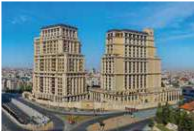
THE RITZ CARLTON HOTEL - AMMAN Sealants
