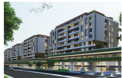
CITY TOWN COMPLEX - SULAYMANIYAH Waterproofing
