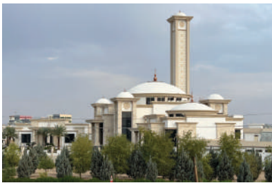
FIRDAWS MOSQUE - ERBIL Waterproofing
