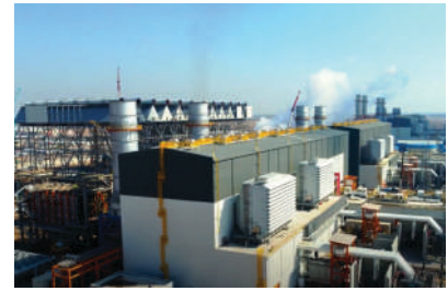
BESMAYA POWER STATION - BAGHDAD Floor coating & sealants
