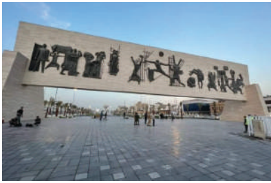
TAHRIR SQUARE - BAGHDAD Waterproofing, concrete repair & tile grouts
