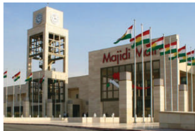
GRAND MAJIDI MALL - ERBIL Waterproofing & sealants
