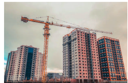
MERSIN TOWERS - DOHUK Waterproofing
