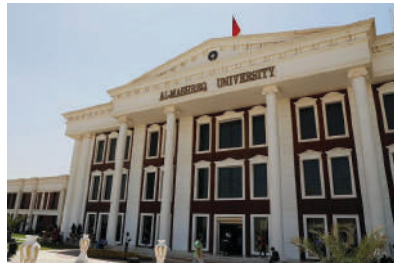
AL MASHREQ UNIVERSITY - BAGHDAD Waterproofing
