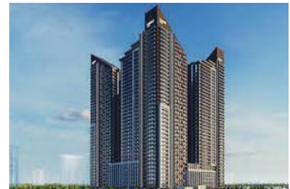
CANDLE KEMPINSKY - ERBIL Waterstops, epoxy anchoring & concrete repair
