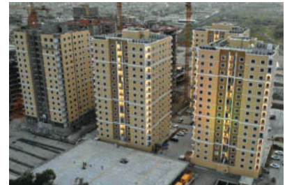
IRAQ GATE COMPLEX - BAGHDAD Waterproofing & sealants
