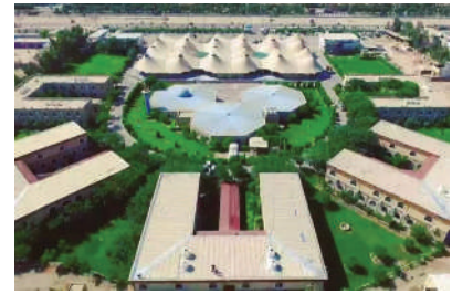
AL AMEED UNIVERSITY - KERBALA Waterproofing, sealants & concrete repair
