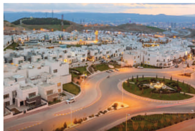
SULI HEIGHTS - SULAYMANIYAH Waterproofing
