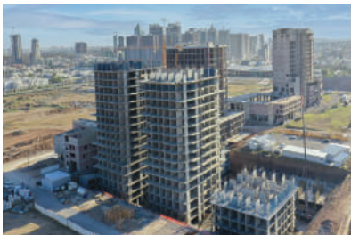
GREEN WORLD - ERBIL Concrete repair, additives & epoxy anchoring
