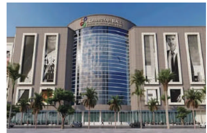
AL AMIRIYAH MALL - BAGHDAD Concrete repair, tile adhesives & sealants
