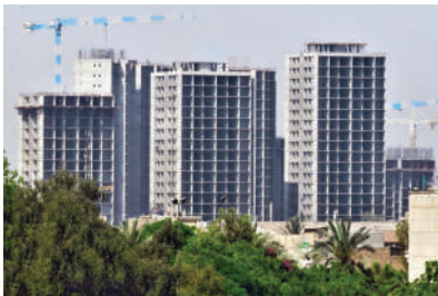
DAR AL SALAM COMPLEX - BAGHDAD Joints, concrete repair & epoxy anchoring
