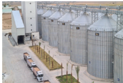
DAS FOOD INDUSTRIES - ERBIL Waterproofing & epoxy coating
