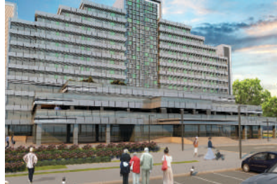
CIHAN HOSPITAL - ERBIL Concrete repair, additives & epoxy anchoring
